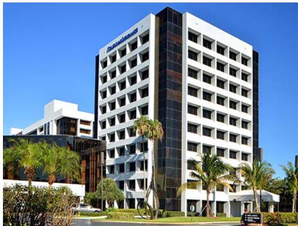
The 10-story office building located at 4400 PGA Blvd. in Palm Beach Gardens, Fla., was 99 percent leased at the time of sale to tenants such as Pulte Homes and the U.S. Army Corps of Engineers.
